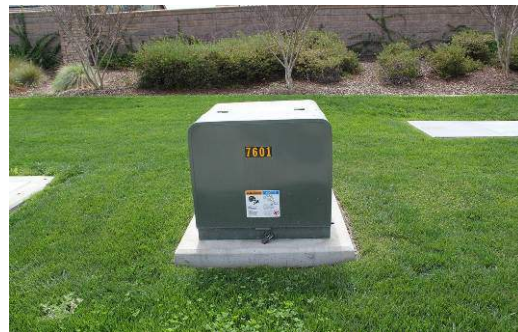
Figure 5 – Single Phase Transformer
